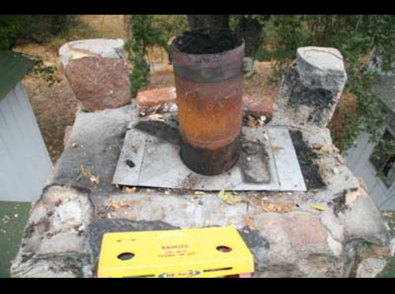
Black steel pipe was used and no weatherproof chase chap. Water ran down the Masonry chimney
